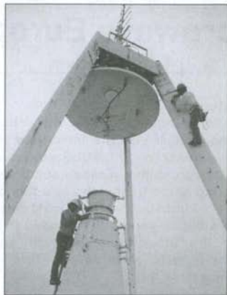
JA1DYB (top) and JE1BNZ (bottom) installing the 4 ele feed Yagis for 2m and 70cm
