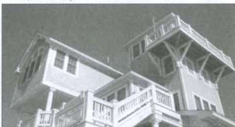
Beacon home with 2m and 6m antenna on roof
